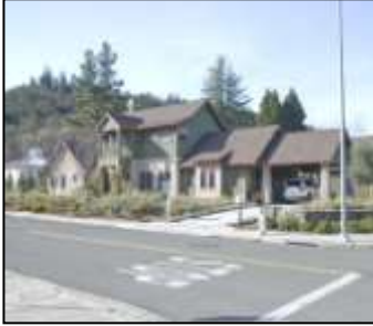
Stop at second house
